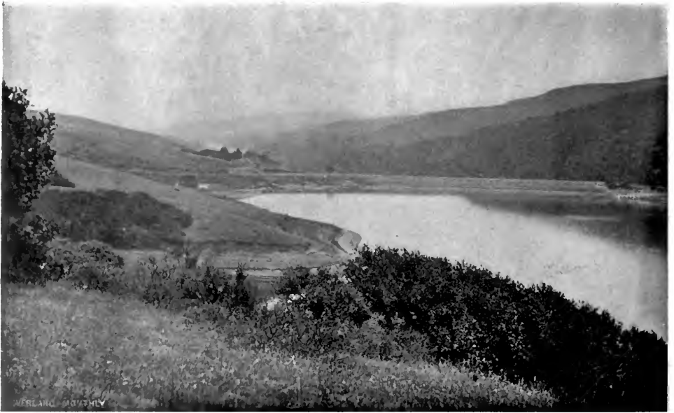
SAN ANDREAS DAM, LOOKING SOUTH.
